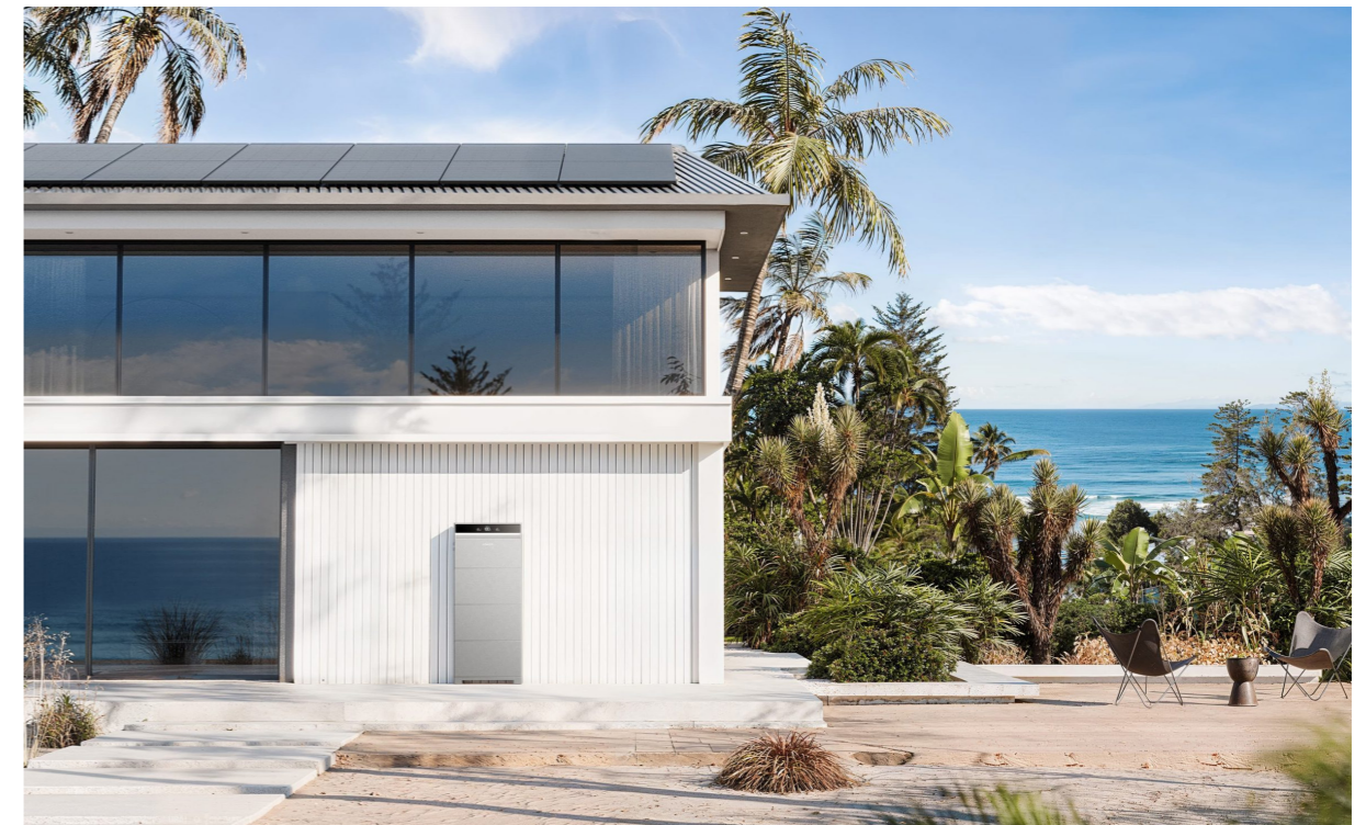
Anker SOLIX × North Kira Australia's First Parallel-Connected SOLIX X1 Home Energy Storage System
